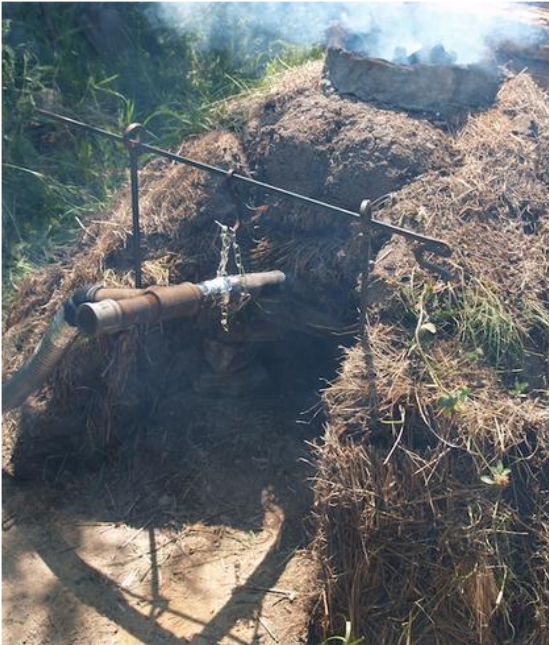
Furnace with air system in place, at first addition of charcoal.
